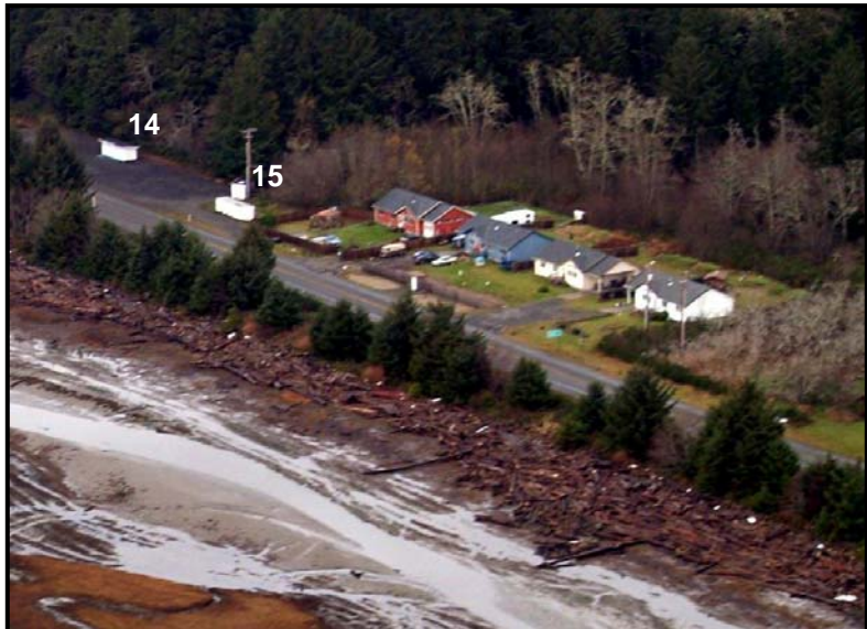
Single Family Residences (Right Side of Photo) (Inventory # 16, 17, 18, 19)
