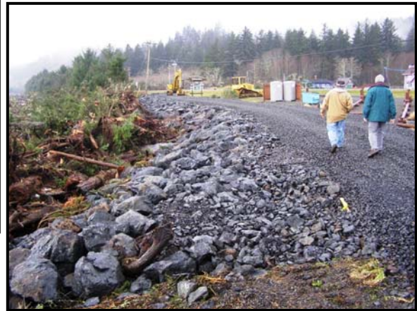
December 2007 flood berm construction, looking east (left photo) and looking west (right photo)
