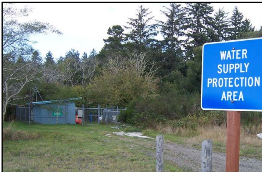
Tribal Water Treatment, Pump House, and Back-up Generator (Inventory # 20)
