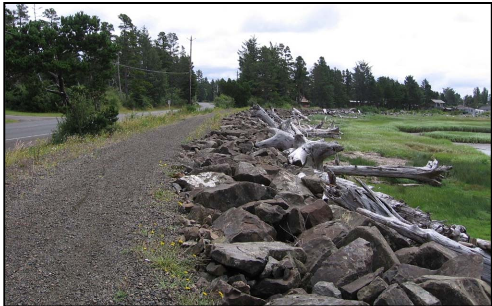
2001 emergency flood berm, looking east
