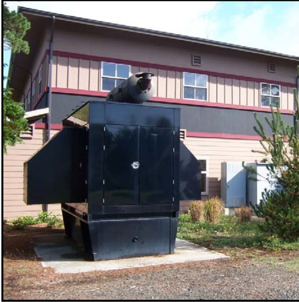
Emergency Backup Generator (Behind Wellness Center) (Inventory # 83a)
