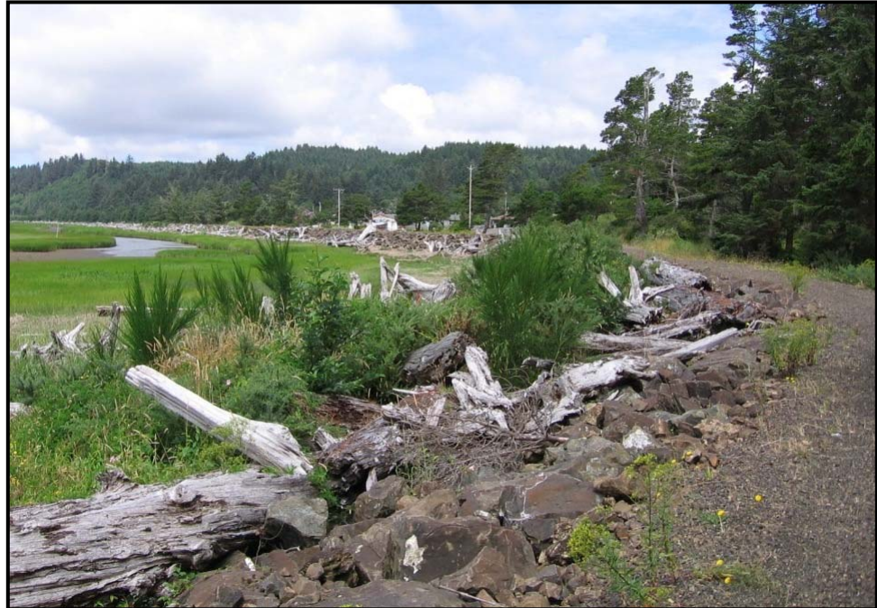
2001 emergency flood berm, looking west
