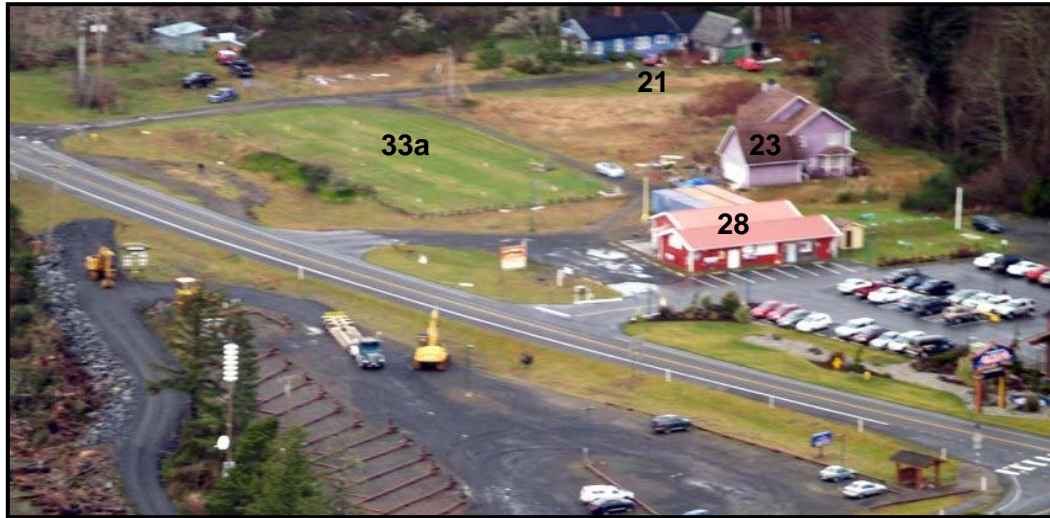
Casino Septic Field, Tribal Business (Convenience Store), and Housing (Inventory # 33a, 28, 21 / 23)
