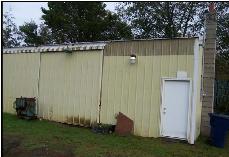
Tribal Warehouse / Maintenance Building (Inventory # 77)
